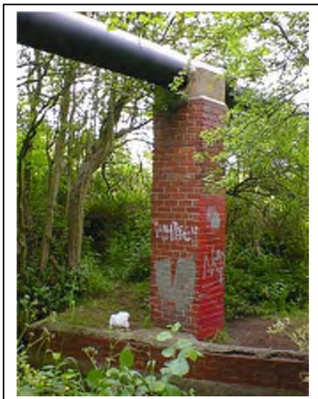
Pipe bridges are more robust structures. Some pipe bridges in addition to pipes carry public footpaths or even vehicular traffic.
