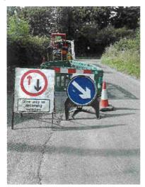
Side protection zones are an essential part of any street works as this provides a buffer zone between the working area and any traffic. The minimum that should be provided is 0.5m
