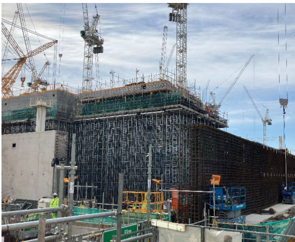
View of the CI Unit 1 Falsework
