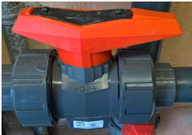
Photo 2: Gas Valve - that should have been fitted.
