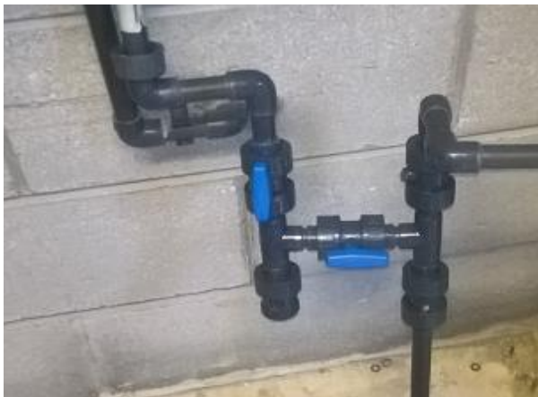
Photo 1: Water Valves - that had been fitted.
