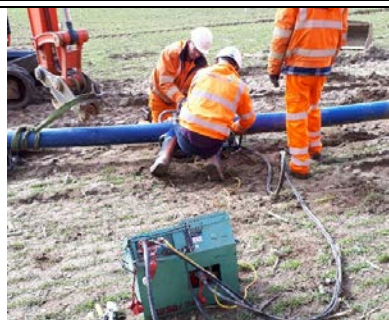
Butt fusion operation on a similar site.
