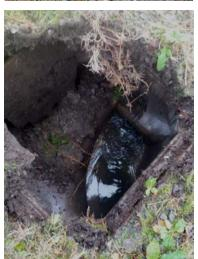
Post incident, the overgrown manhole cover was dug out of the ground, the drain top and recess were cleaned out and the manhole cover was placed over the chamber. There was no apparent reason for the cover to have been removed and to have been replaced by a temporary wooden board.
