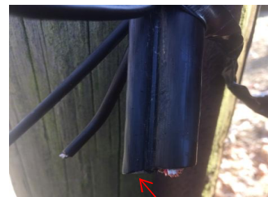
BT Main cable with steel section
