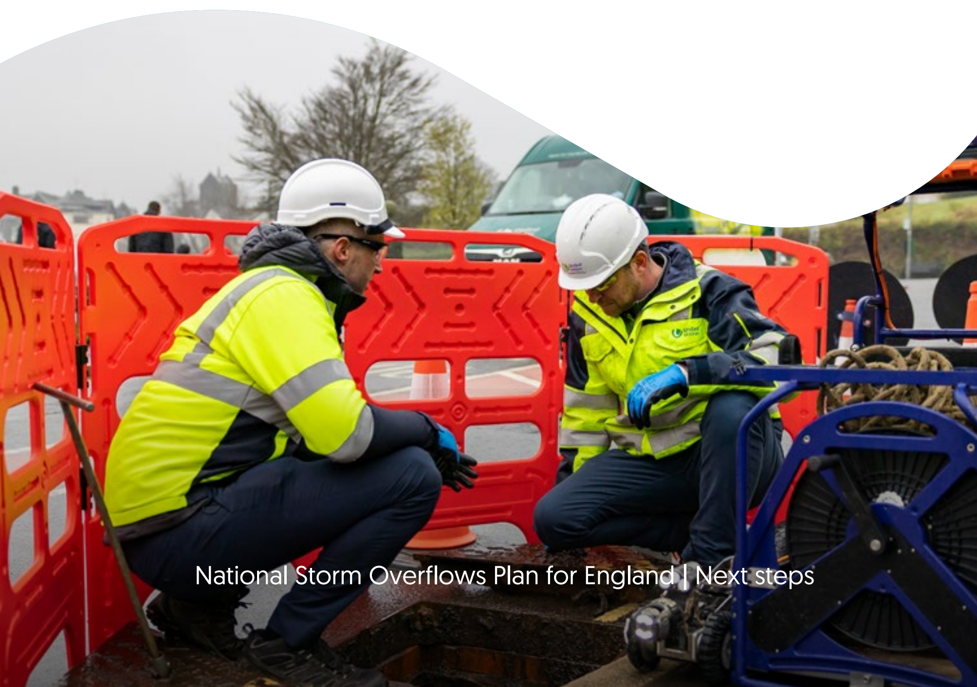
Image: Work on a smart sewer
