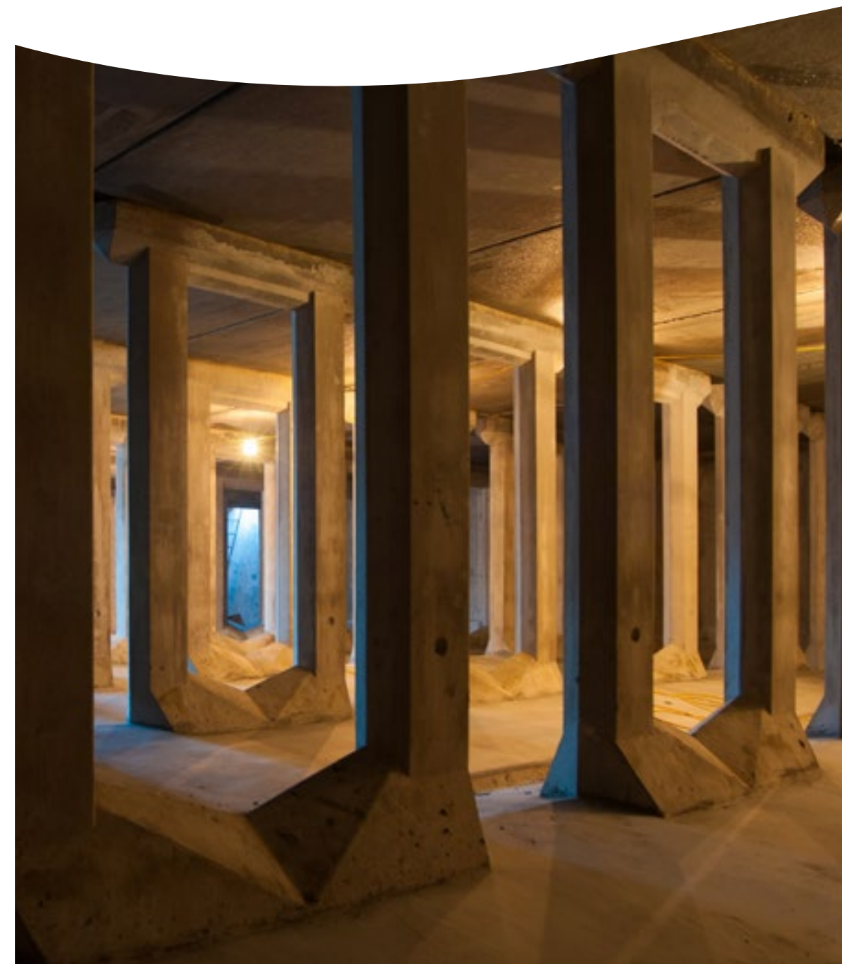
An example of scale: The size of several Olympic-sized swimming pools in volume, this image shows a typical storage tank.
